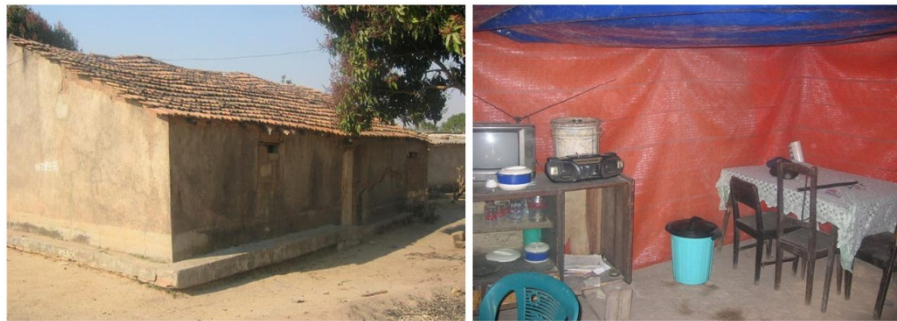
Figure 1 Cacilhas, Huambo Province, Angola. Sixty households (left) in an urban area of Huambo Province, Angola, received a polyethylene shade cloth durable lining (DL) and a heavy-weight insecticide-treated plastic sheeting (ITPS) to cover the walls and ceilings of their houses, respectively (right).
