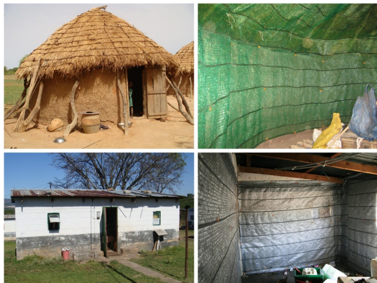
Figure 3 Durable linings (right) installed in traditional houses in rural Mali (top left) and South Africa (bottom left).
